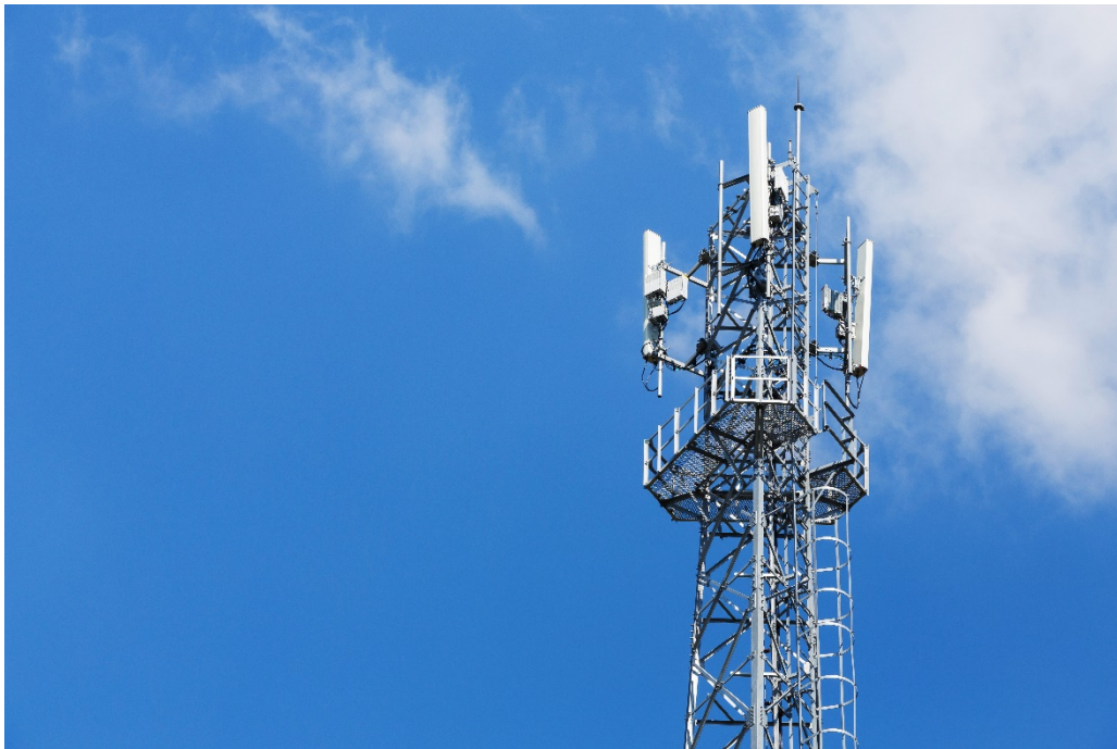
Fig 1.2.16: Connection of a repeater in an antenna for transmission of information
